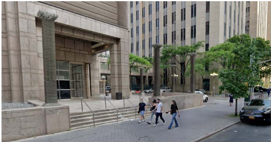
VIEW FROM CENTRE ST LOOKING SOUTH-EAST
