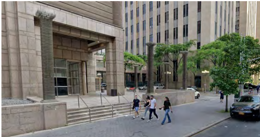
VIEW FROM CENTRE ST LOOKING SOUTH-EAST
