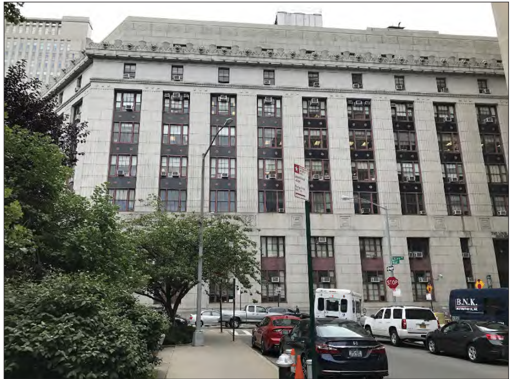
View southwest of the north façade of the Louis J. Lefkowitz State Office Building along Baxter Street
