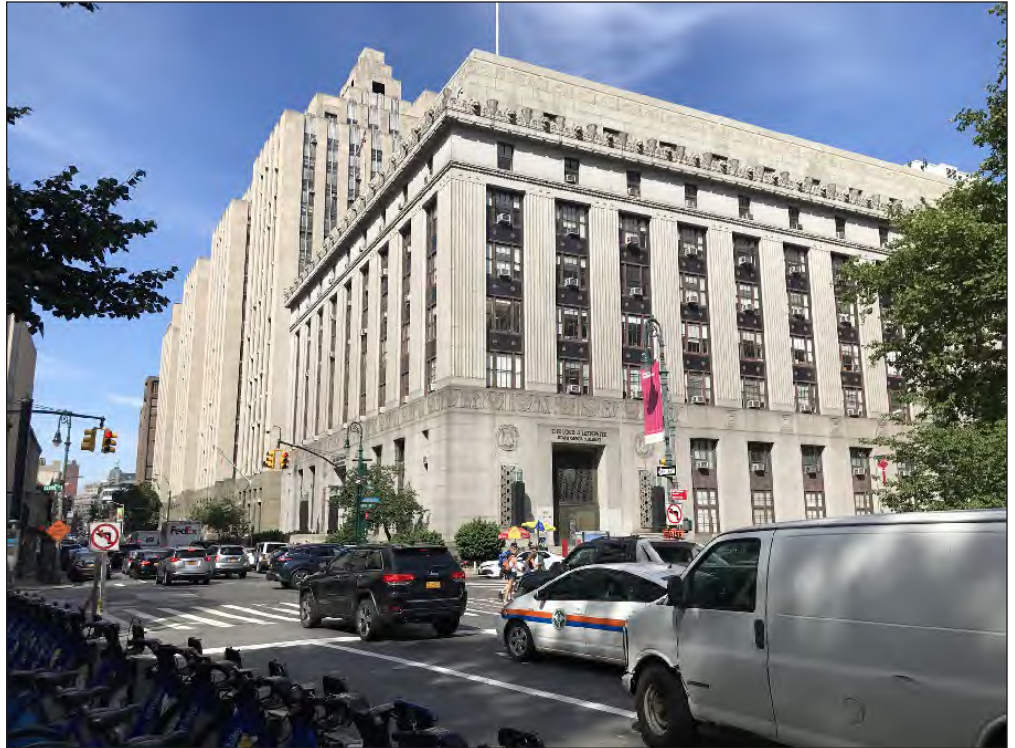
View northeast of the Louis J. Lefkowitz State Office Building from Centre Street south of Worth Street
