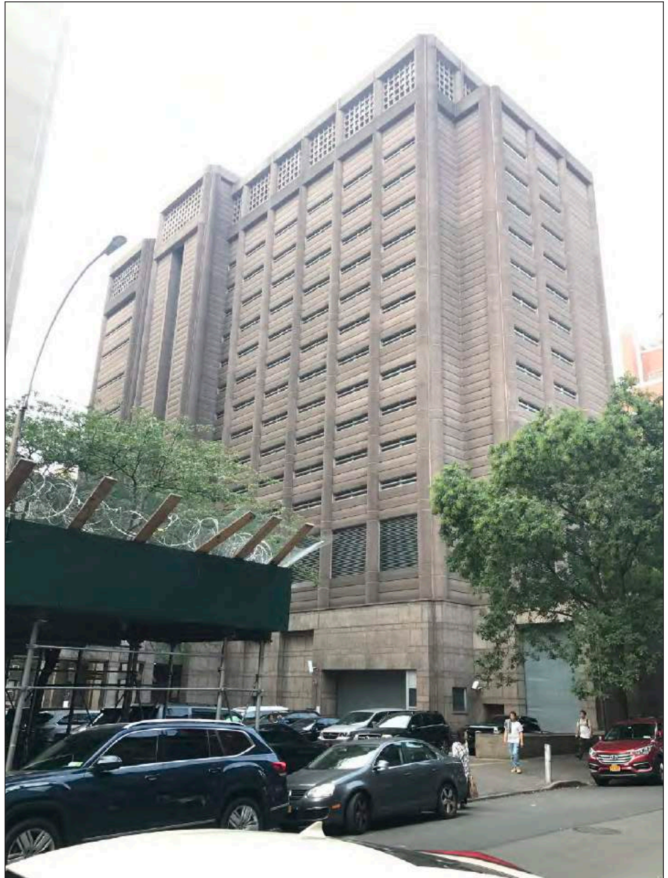
View northwest from Baxter Street of the North Tower of the Manhattan Detention Center at 124 White Street (Block 198, Lot 1) 3
