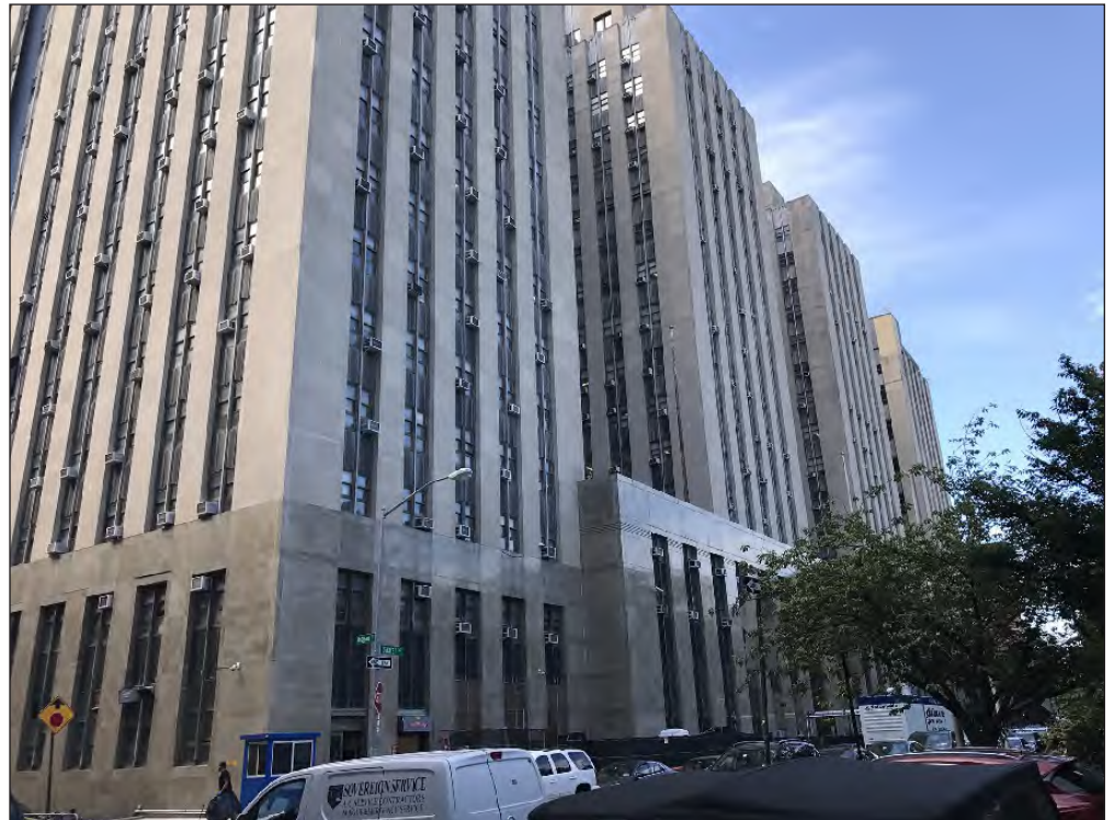
View north along Baxter Street of the Criminal Courts Building and Prison building from Hogan Place 5
