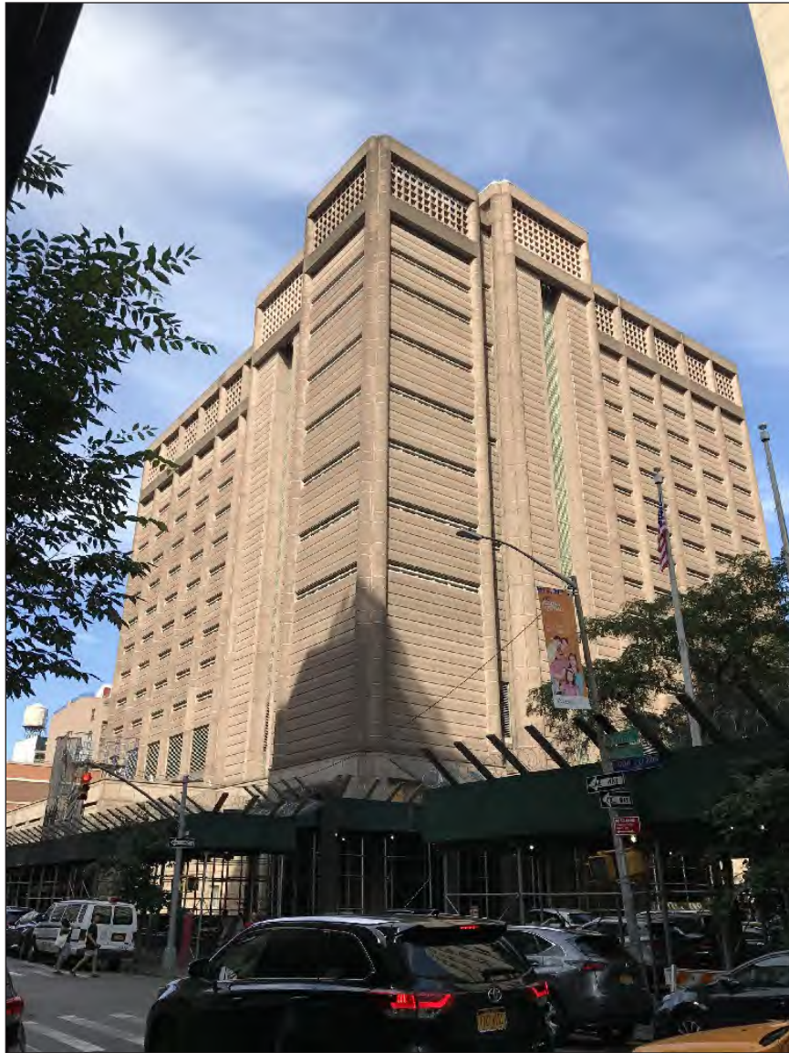
Northwest view of the project site from Centre Street, showing the south and west façades of the North Tower 3
