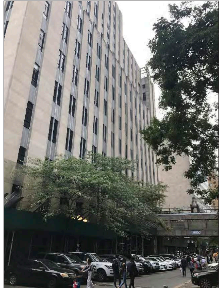
View southwest from Baxter Street of the north façade of 125 White Street
