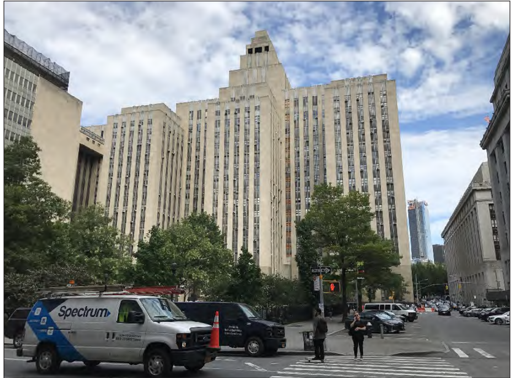
View east along Leonard Street of the Criminal Courts Building and Prison building (NYCL-eligible, S/NR-eligible) at 100 Centre Street (Block 167, Lot 1) 4
