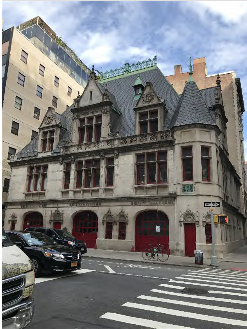
View east from White Street of the Fire Engine Company No. 3 building (NYCL, S/NR-listed) at 87 Lafayette Street (Block 197, Lot 1) 12
