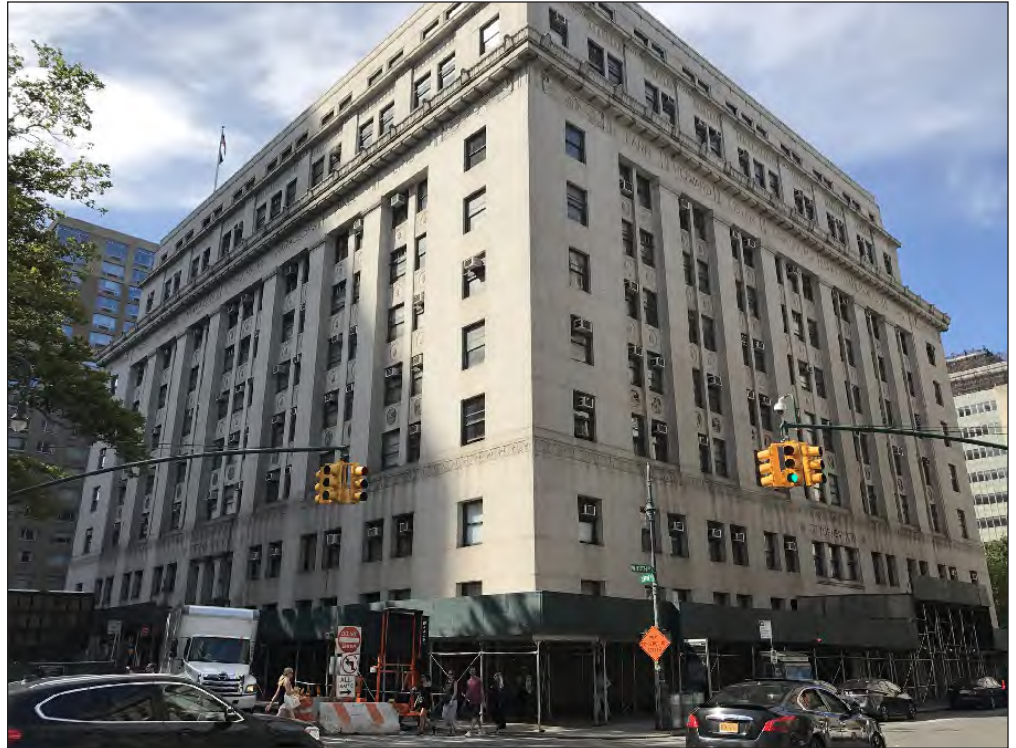
View northwest of the City of New York Building (S/NR-eligible) at 75 Centre Street 10 (Block 168, Lot 32) from the southeast corner of Centre and Worth Streets
