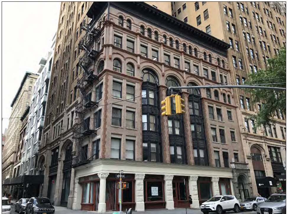
The Ahrens Building (NYCL, S/NR-eligible) at 70-76 Lafayette Street (Block 172, Lot 23)
