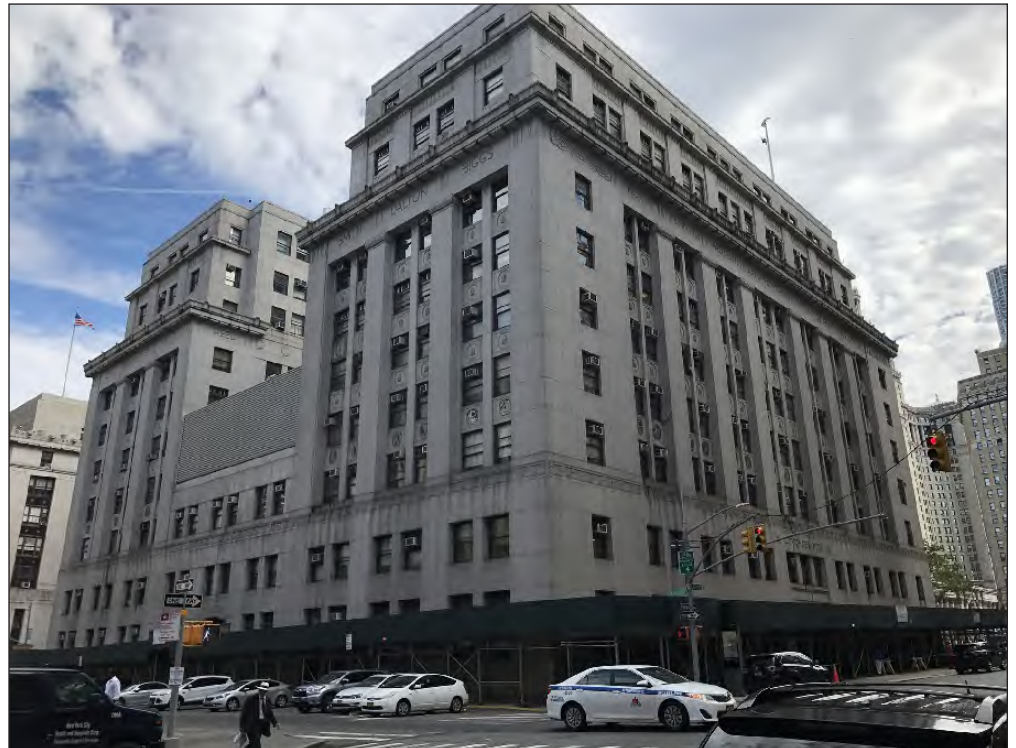
View southeast of the City of New York Building from the intersection of Lafayette and 11 Leonard Streets
