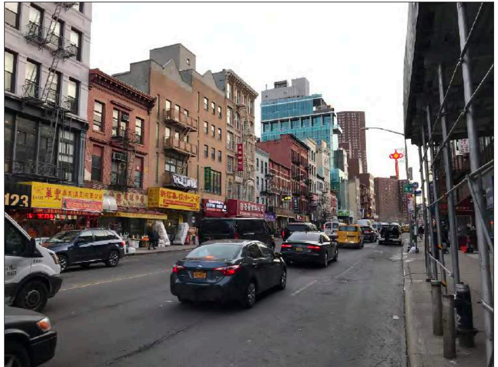
View south on Bowery, showing the 18-story contemporary hotel in the distance 40
