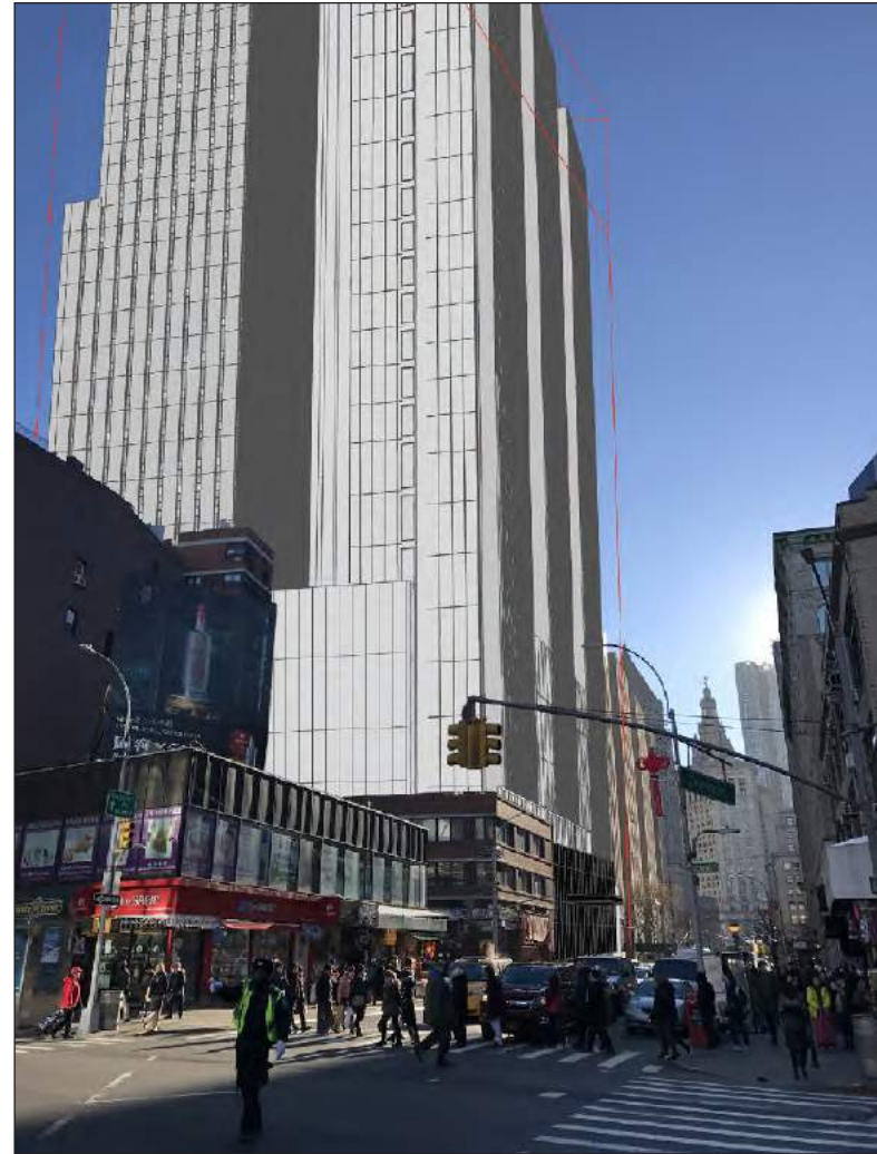
View south from Centre Street and Canal Street
