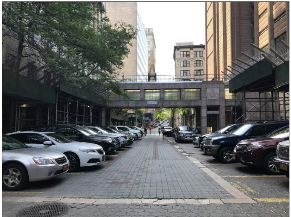
West view of the Manhattan Detention Complex on White Street, currently used for parking and as entries to the North and South Towers, and pedestrian bridge connecting the North and South Towers
