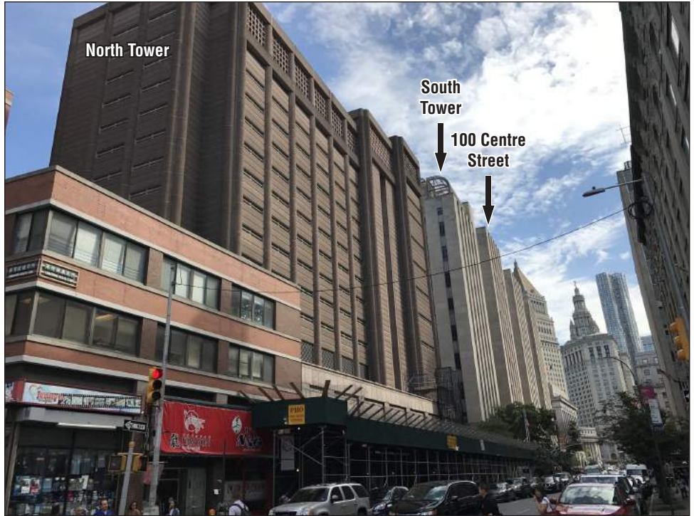
South view of the Manhattan Detention Complex on Centre Street, showing the existing North Tower and the South Tower on the east side of Centre Street
