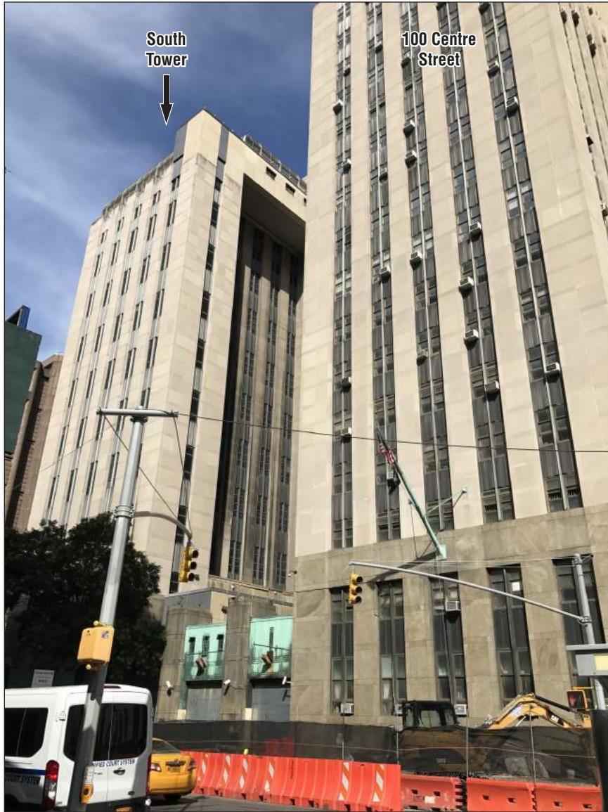
Northeast view of the Manhattan Detention Complex from Centre Street, showing the west façade of the South Tower, the sallyport entrance and a portion of 100 Centre Street
