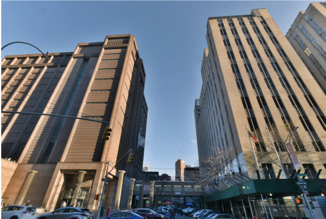
Under the city's plan, the north and south towers of the Manhattan Detention Center (24 White Street, right, and 125 White Street) would be demolished and replaced by a jail as tall as 50 stories. Photo: Carl Glassman/Tribeca Trib
